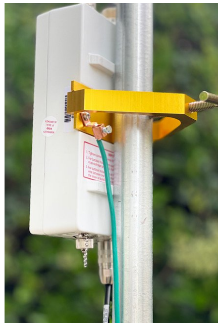
Figure 3.3 - pulsedAR radio mounted on a pole
